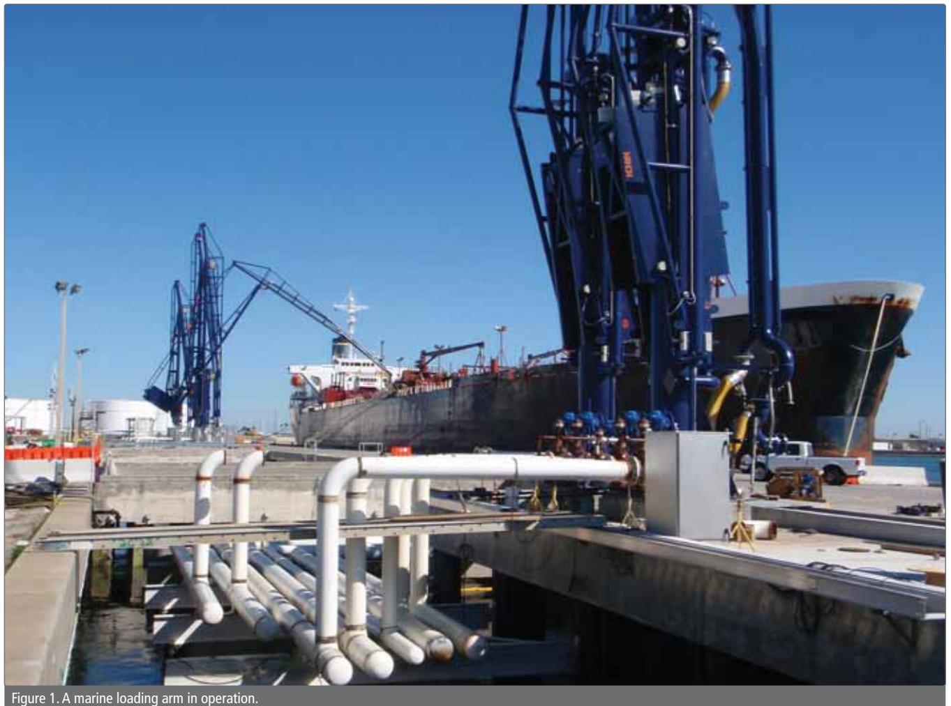
Figure 1. A marine loading arm in operation.
